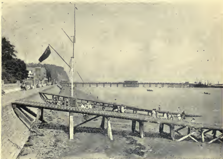
The Pier, Penarth.
