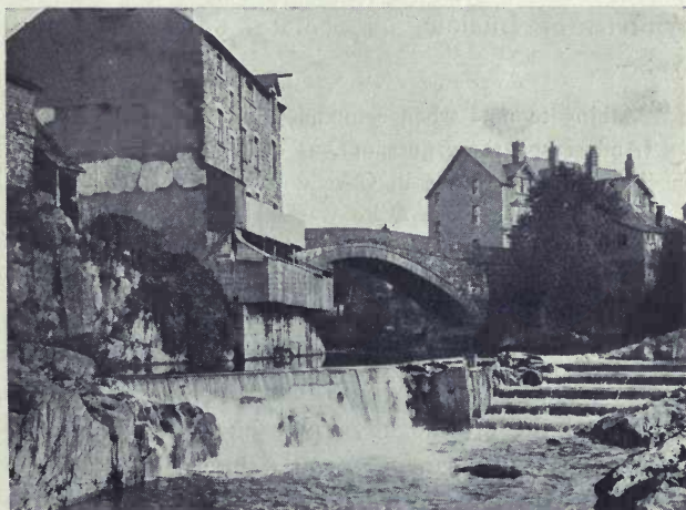
Salmon Ladder, Rhayader Bridge
