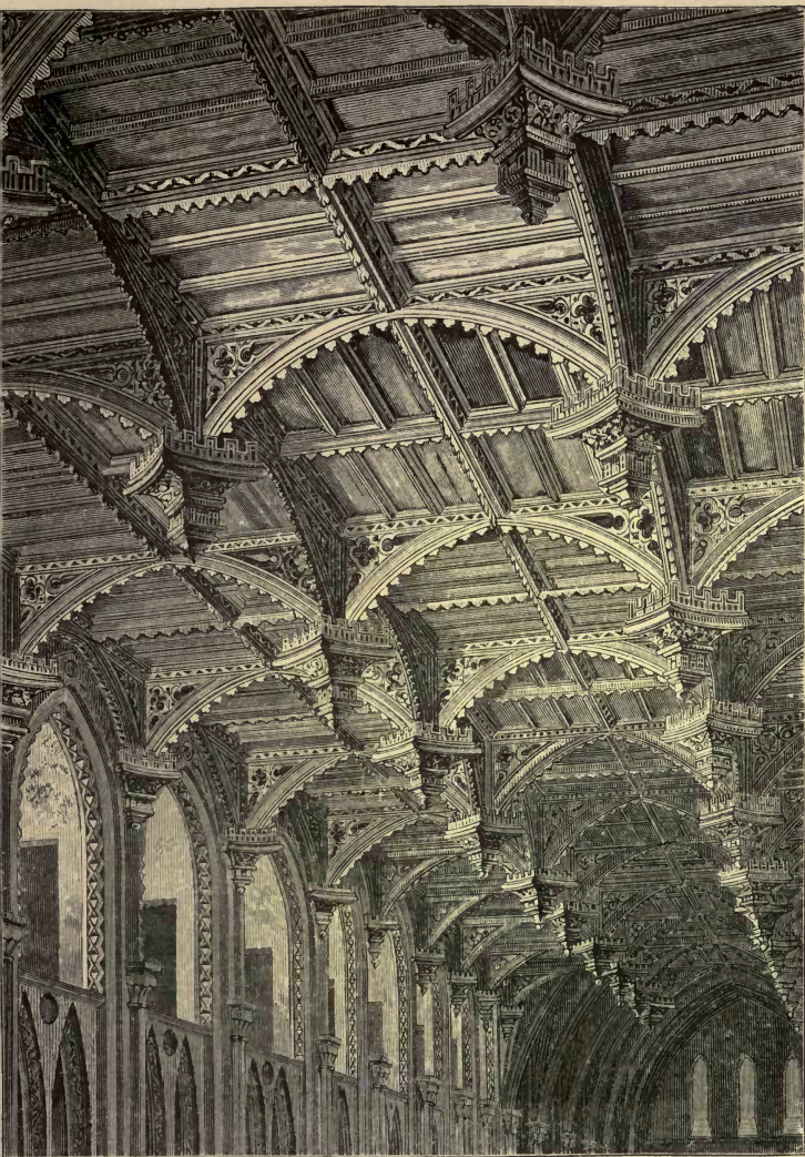
ST. DAVID'S CATHEDRAL. ROOF OF NAVE.
