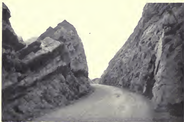
Cutting on the road near the Mumbles
