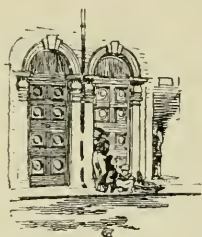
DOORWAYS, CRAMPTON COURT
