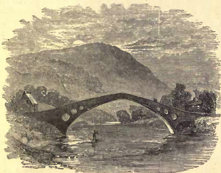
PONTYPRIDD BRIDGE: W. EDWARDS, BUILDER, 1755.
