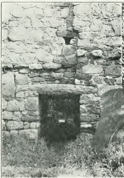
West Doorway of the Ruined Church of Dalkey.
