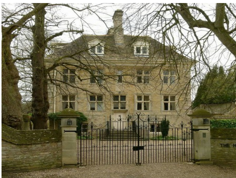
South Luffenham Hall
